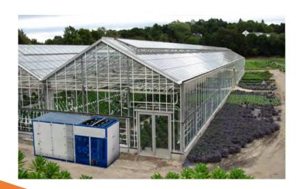
**AWA systems**, integrated with greenhouses, allow to control the internal humidity producing pure water to be used for irrigation or other agricultural purposes.
